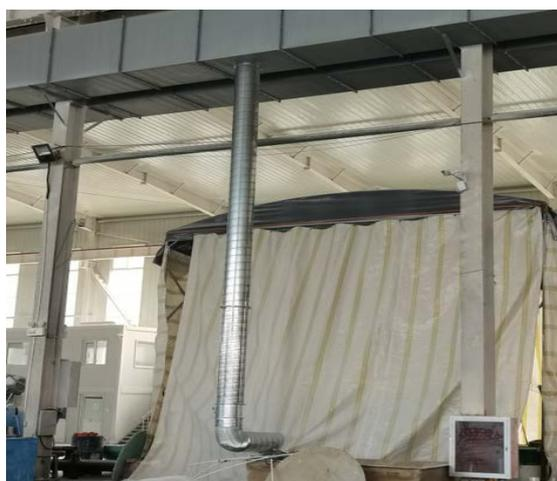
3 号车间切割工序二次密闭连接集气罩
