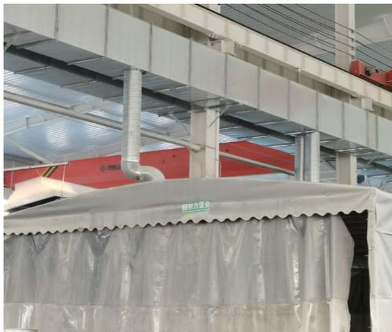
7 号车间切割工序二次密闭连接集气罩
